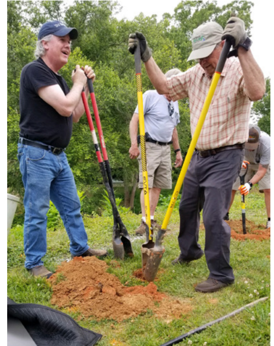
Doug Mitchell and William Blackley install the new interpretive sign. Photo courtesy William Blackley.
